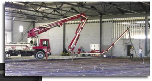
multaneously with boom unfolding to further speed concrete placement. The patented Auto-Scissors pipeline adjusts to all boom positions without exceeding overall height for reliable delivery of concrete to the end hose.
